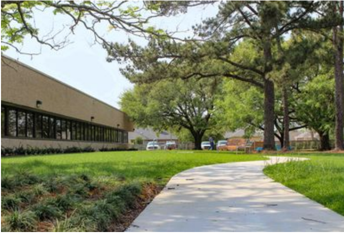
side of building 1
