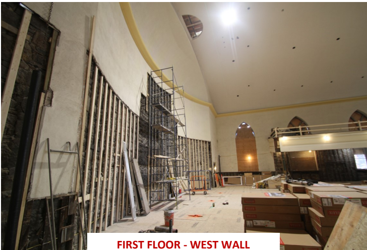
FIRST FLOOR - WEST WALL
