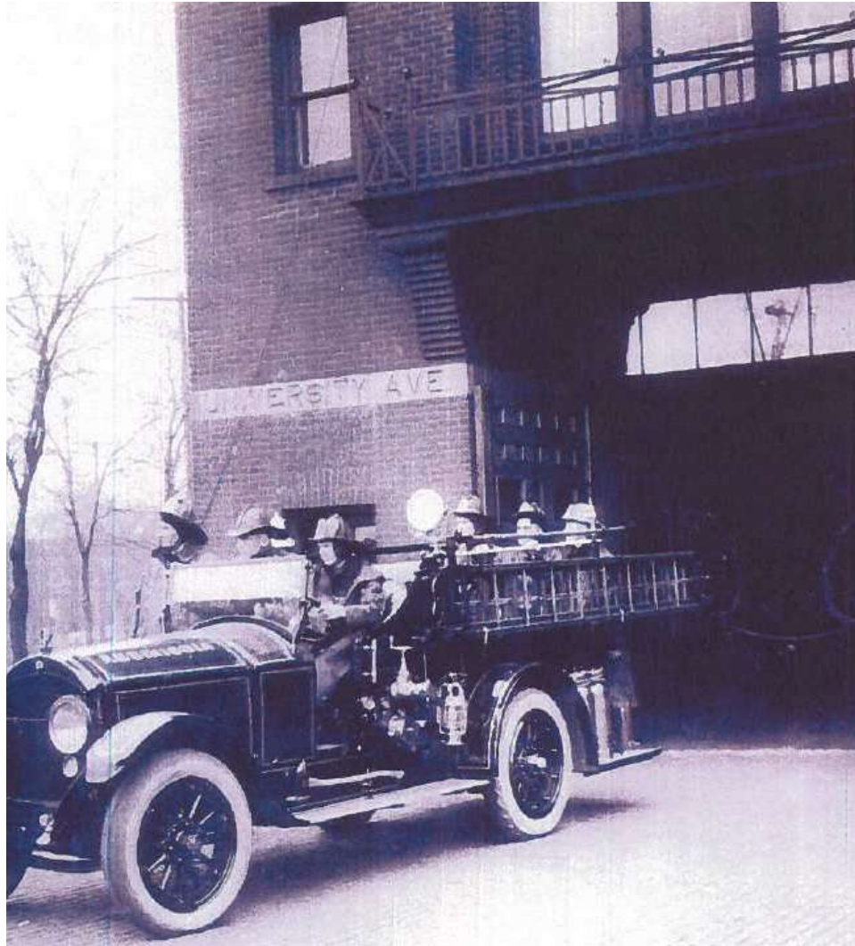
Station 19 Firehouse - 1920's
