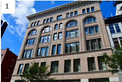
1 THE BANKERS ALLEY HOTEL Opened August 1, 2023 124 Rooms Gray & Dudley 1st floor art museum 222 3rd Ave N
